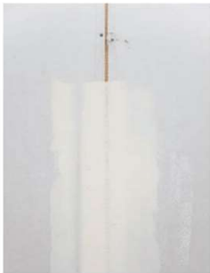
4 This first application flattens the tape and also provides a level base for the subsequent layers of filler.
